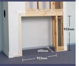
Zero Clearance Box positioned in framework on 12mm sheet
